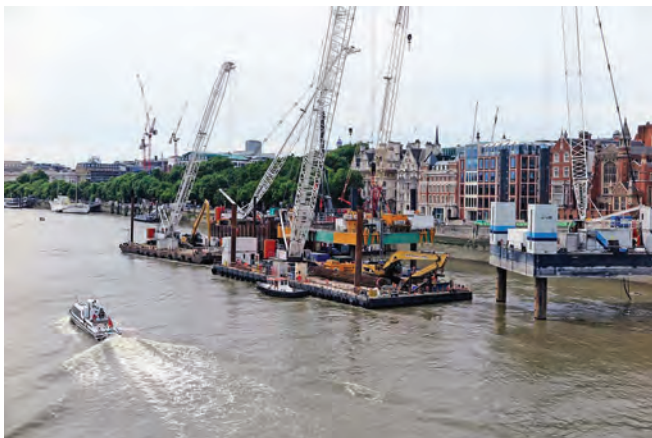
Coffer dam at Blackfriars Bridge Foreshore
